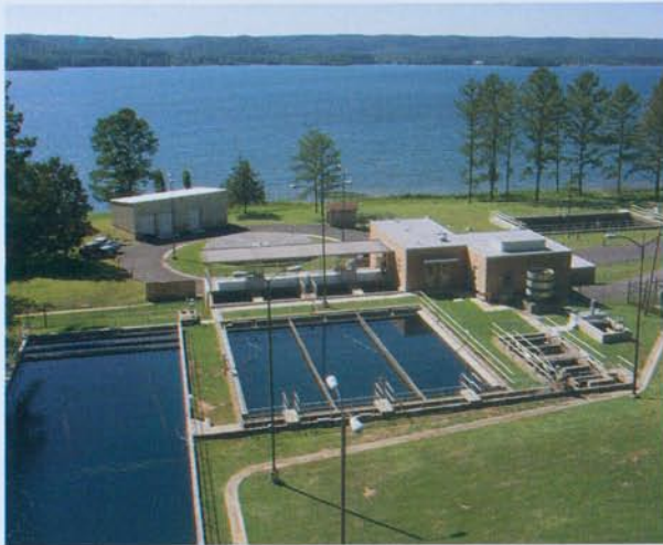
Sunset Water Treatment Plant on beautiful Lake Guntersville
